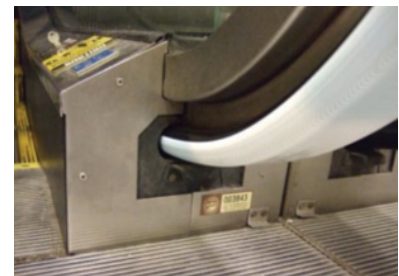
Photo 10 - Inlet Inspection
